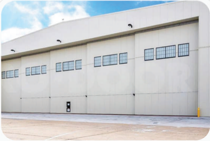
Sliding Aircraft Hangar Doors
