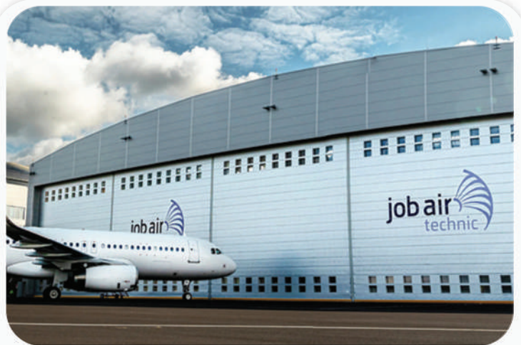
Lifting Aircraft Hangar Doors
